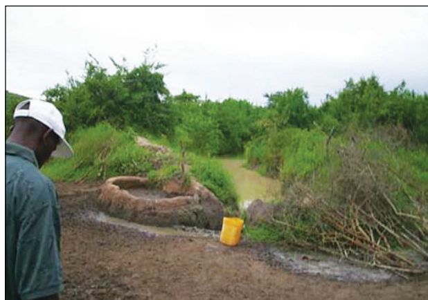
Watering troughs molded out of clay to prevent animals drinking directly from water reservoir and also used for domestic water, Kazo-Mabarara. Photo credit: David C. Waiswa
