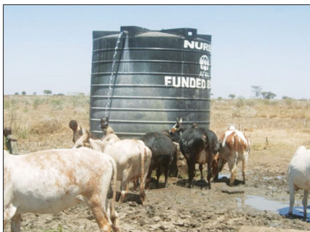
Water pumped from a valley dam into a reservoir tank to facilitate watering animals, Karamoja. Photo credit: Daniel Aleper
