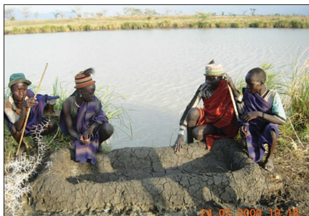
Valley dam with earth-molded drinking trough constructed by water committee to prevent animals drinking from reservoir, Karamoja. Photo credit: Daniel Aleper
