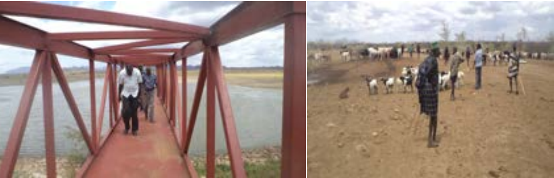
Figure 1: On the left, reduced water levels in Kobebe dam in Moroto districts. The dam has not dried up for over 3 years and has been handy during the prolonged dry spells in Karamoja although levels went abnormally low in 2016. On the right, the Matheniko and Turkana animals congregate in Kobebe to drink water.
